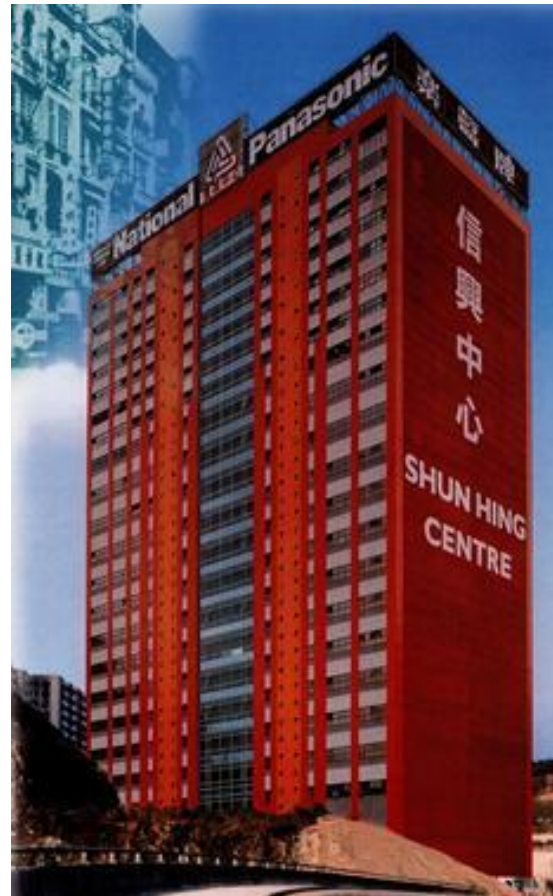
Hong Kong Shun Hing Centre
